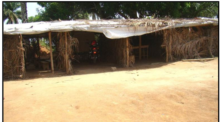
An existing school structure.
